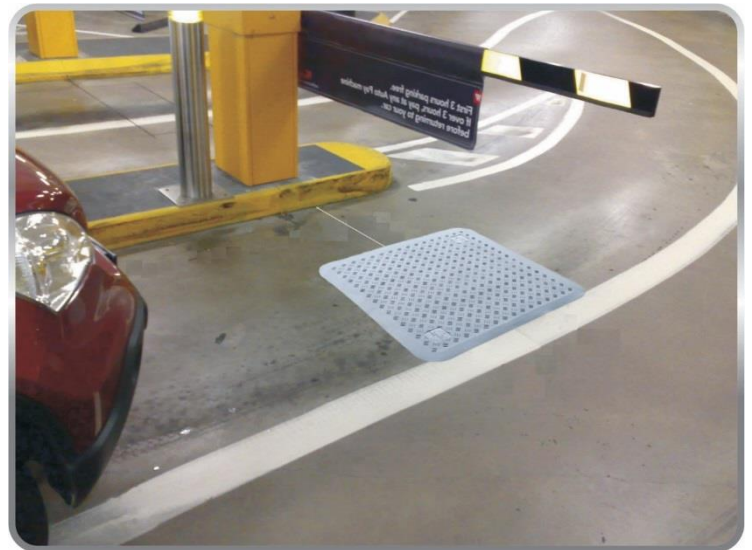
New SMR-900 utilising existing Lead Wire slot
